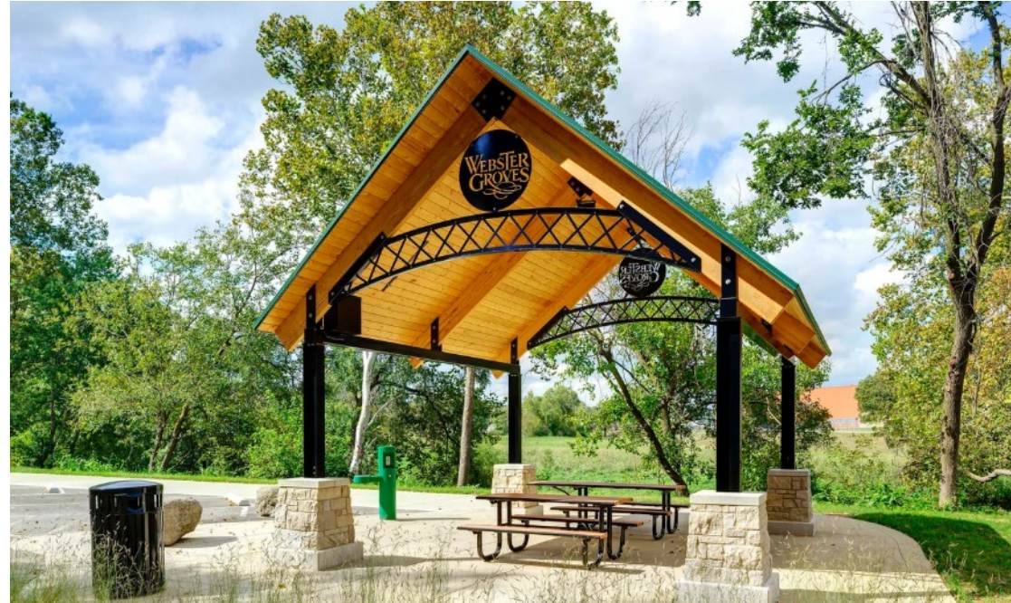
Gable Roof With Steel Post and Glulam Beams
