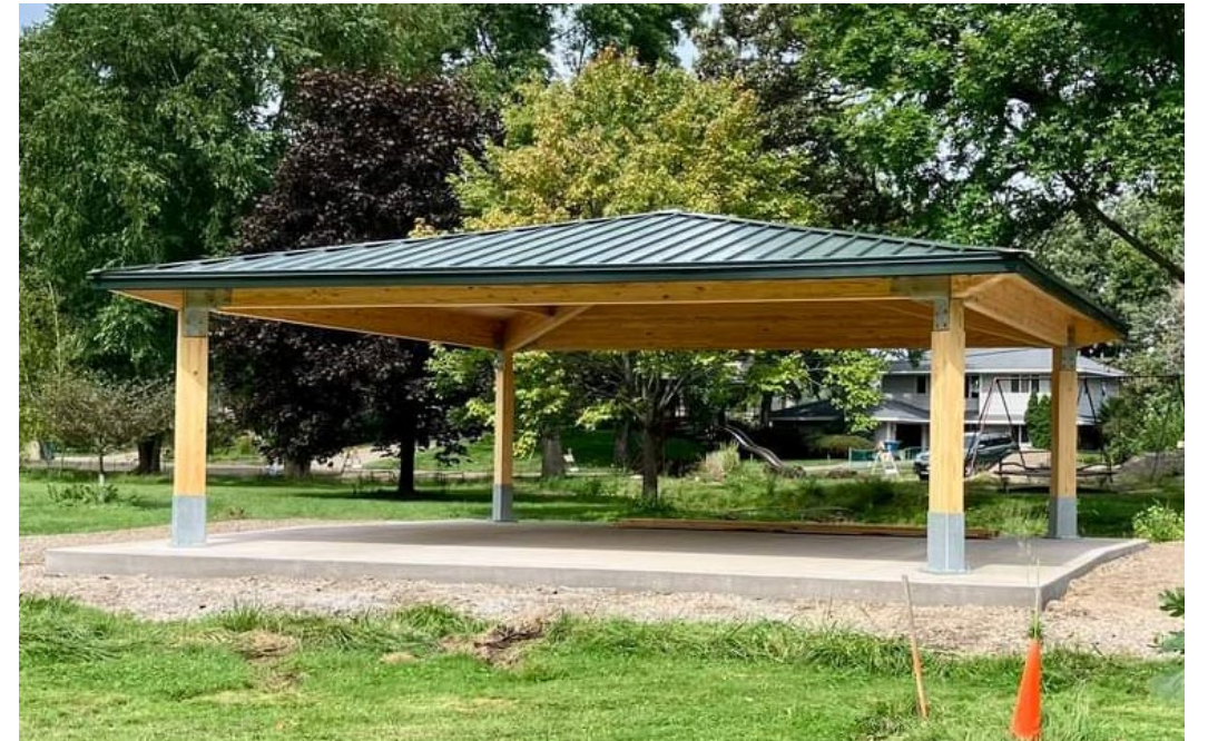
Hip Roof with Glulam Posts and Beams
