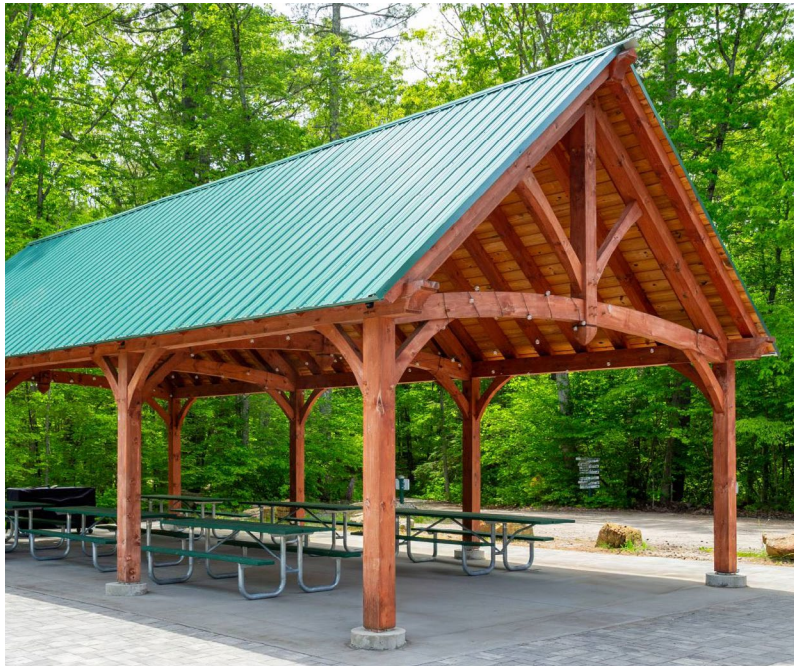
Gable Roof with Timber Frame
