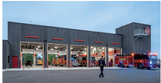
Lake Elmo Public Facilities, City Hall and Fire Rescue
