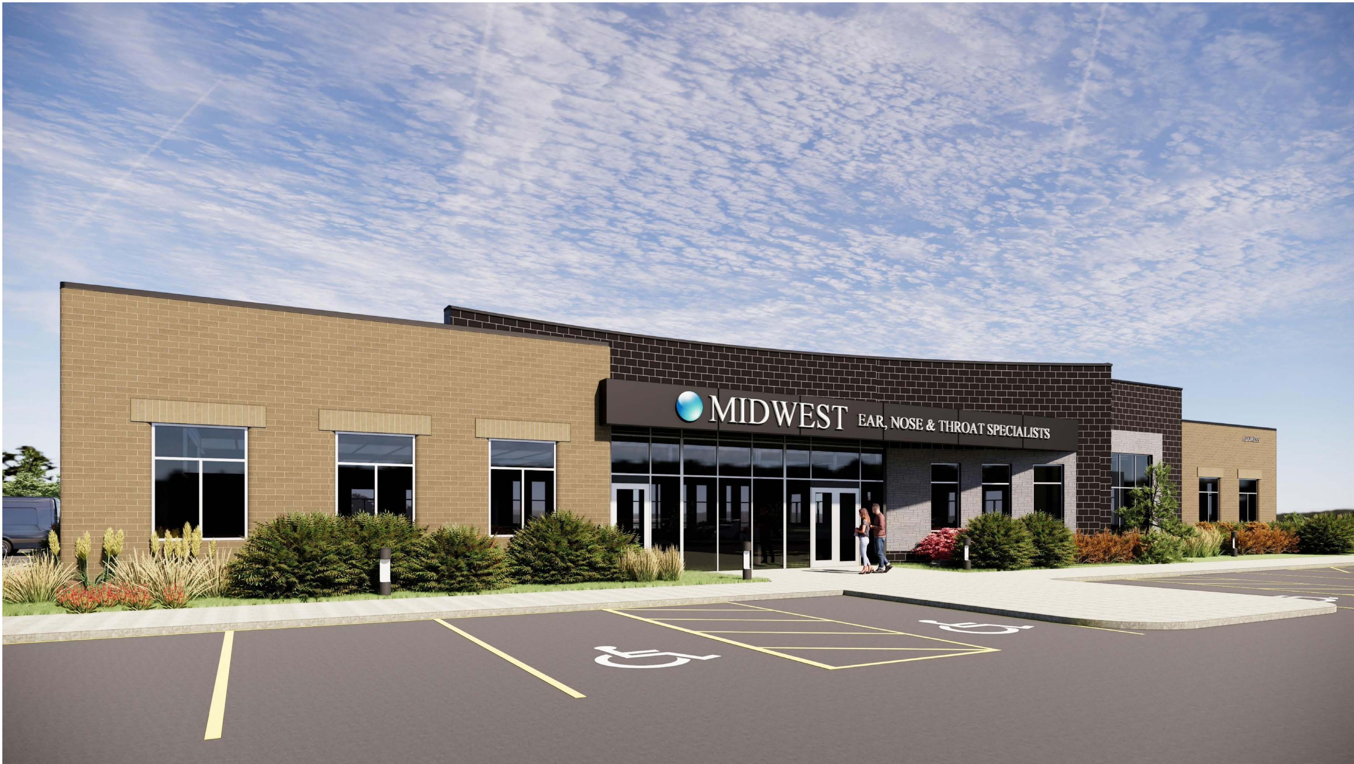
BUILDING ENTRY ( WEST)
