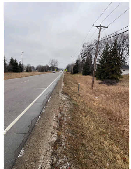
▲ Overhead power lines on the east side of Dodd Boulevard will be a key consideration as alternatives are evaluated.
