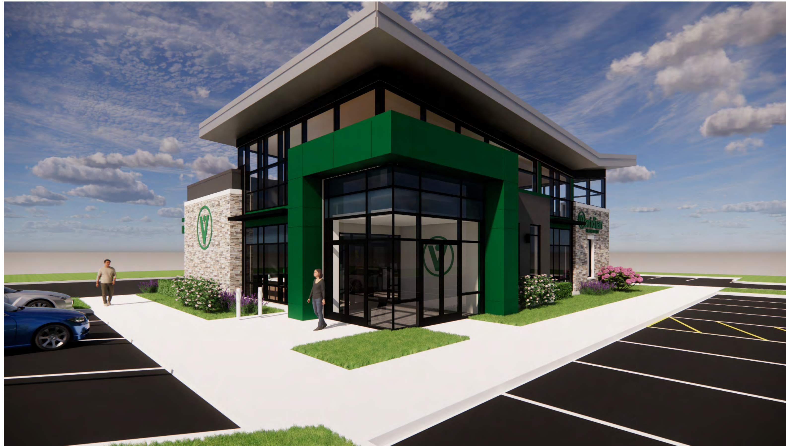
Building Entrance (Day): Green Alpolc metal panels frame the aluminum glass system. Carbon colored aluminum siding breaks up overall facade. A stone blend anchors the corner of the building as well as provides an area for signage.
