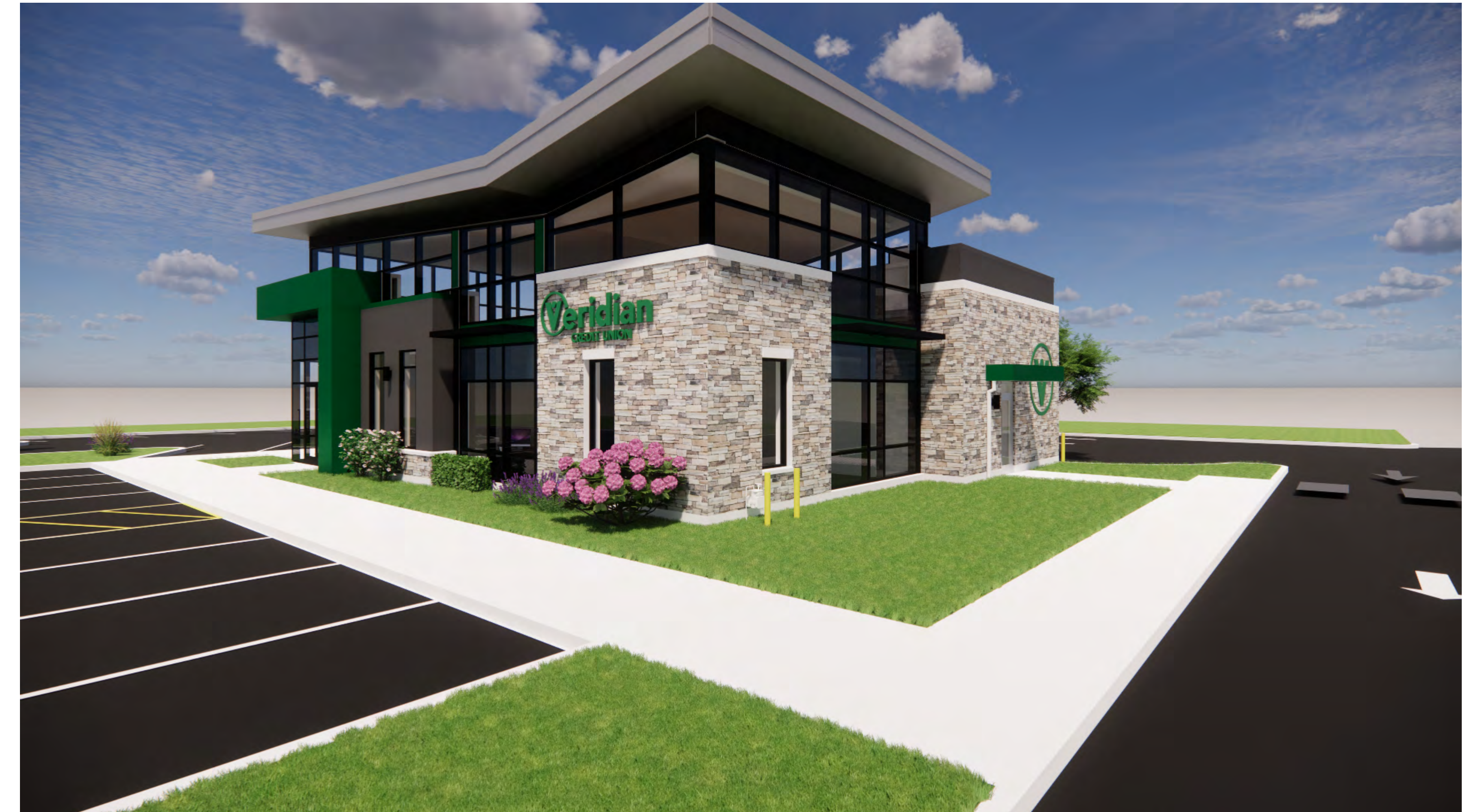
Southwest Elevation: The carbon colored aluminum siding frames a natural stone blend that is used across the elevation, broken by clearstory windows that provide natural light to the Teller Work Area. Back-lit signage is also used on the west elevation. Green LED tape light is placed at the top of the stone band which provides additional branding and visual interest to the building at night.
