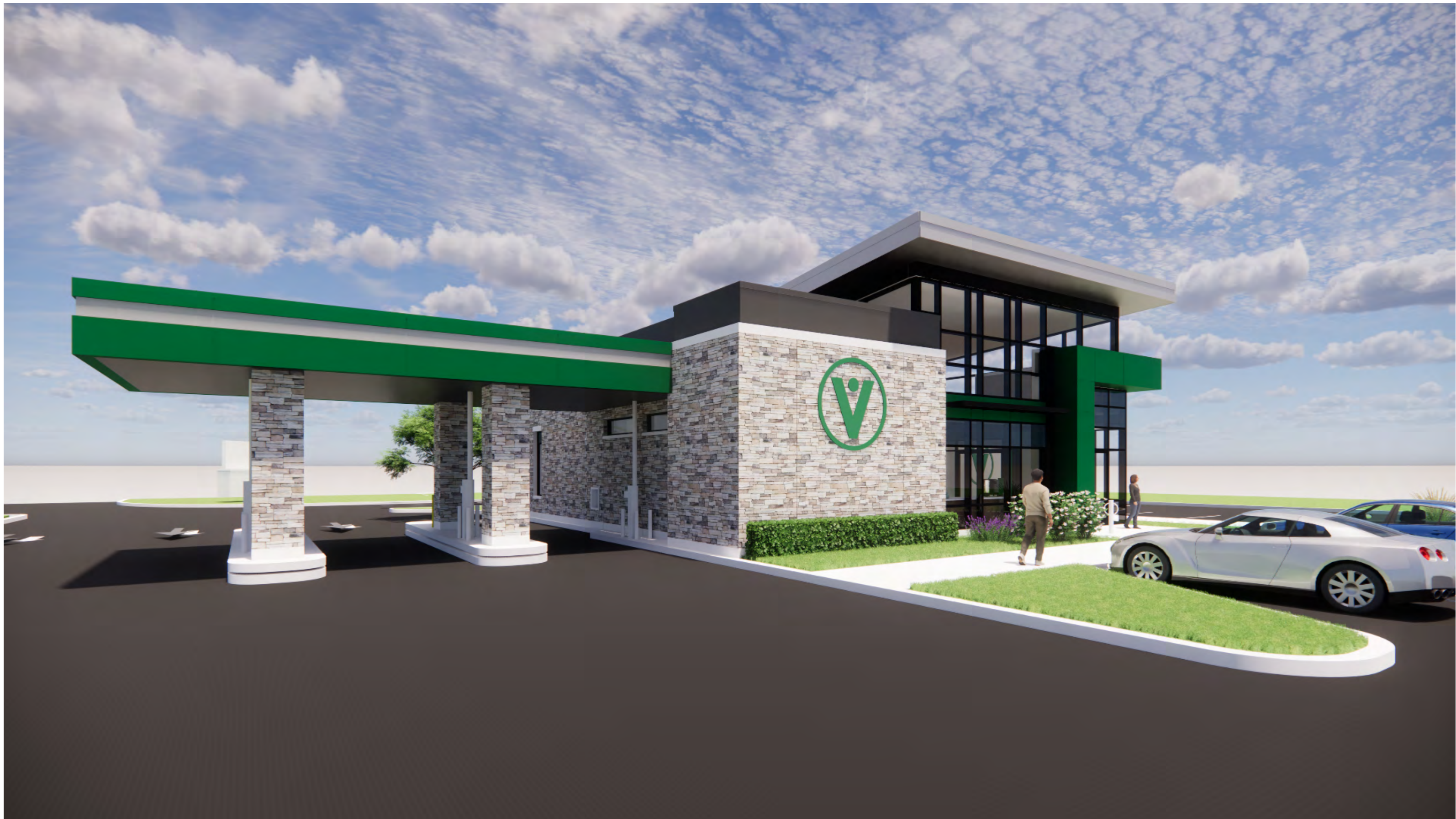
Drive-Up Canopy: Green Alpolic metal panels continue to pull the Veridian marketing colors onto the north elevation. The canopy will contain the pneumatic tubes as well as can light fixtures as well as green tape lights along the interior edge for nighttime lighting.
