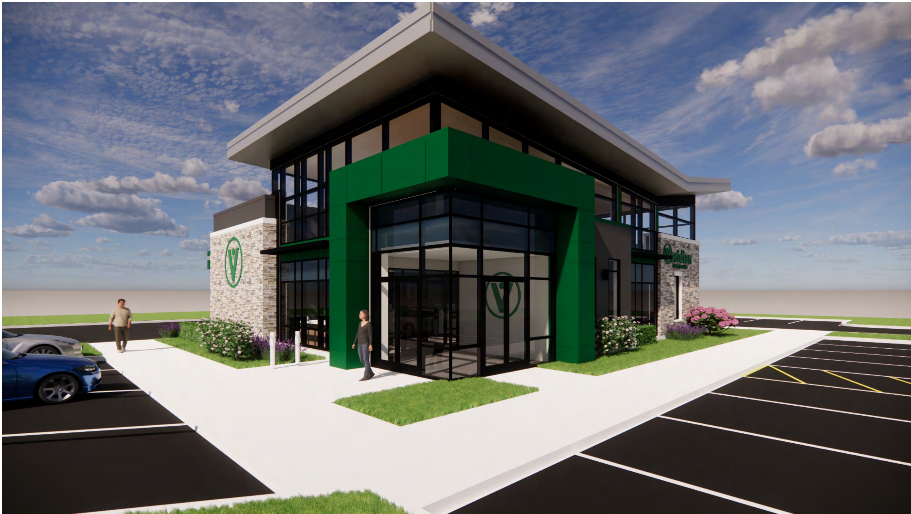
Building Entrance (Day): Green Alpolic metal panels frame the aluminum glass system. Carbon colored aluminum siding breaks up overall facade. A stone blend anchors the corner of the building as well as provides an area for signage.
